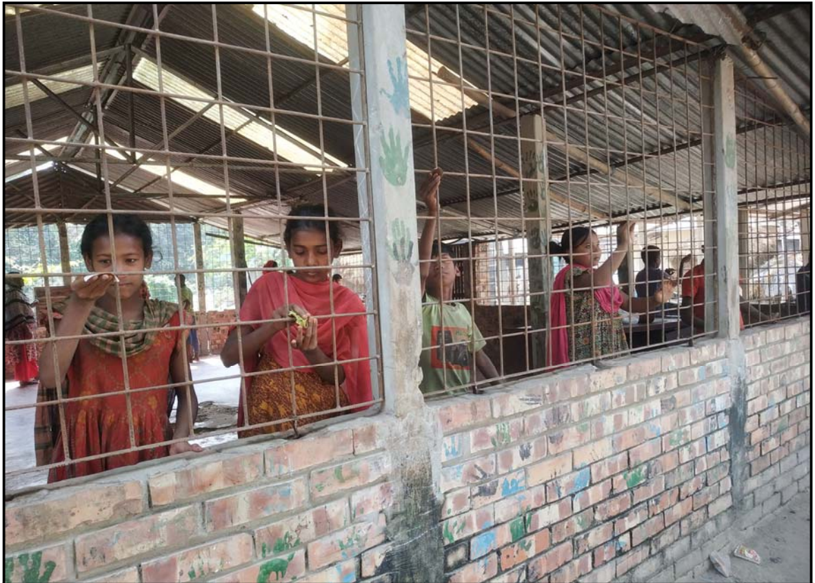
To avoid rust of the school grills all students clean it with sandpaper...
