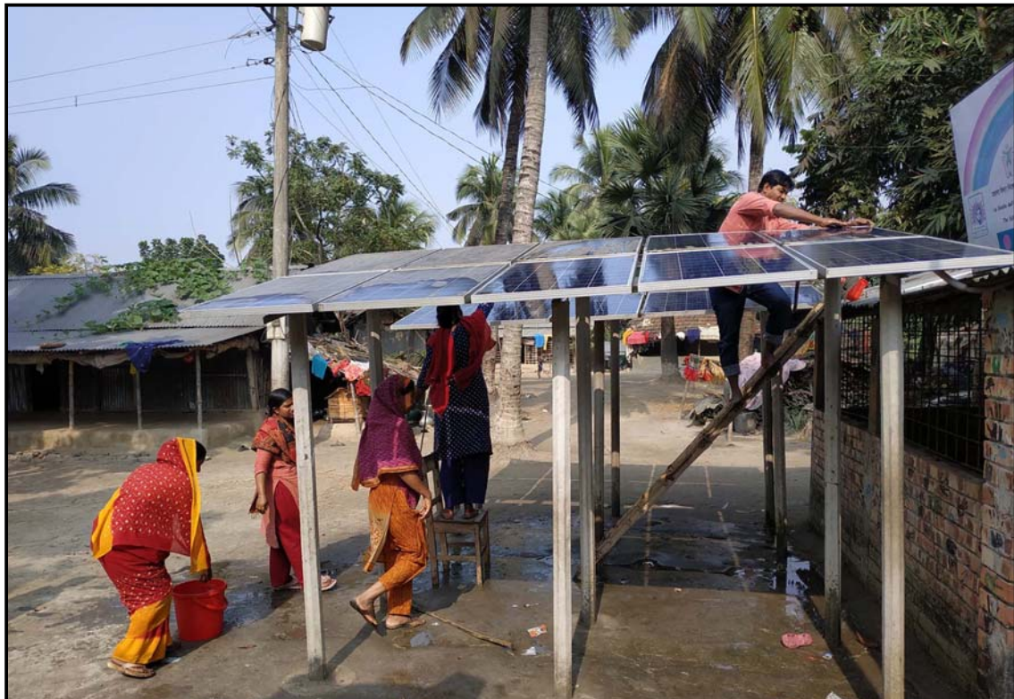
Solar Water Pump maintenance by teachers and villagers...
