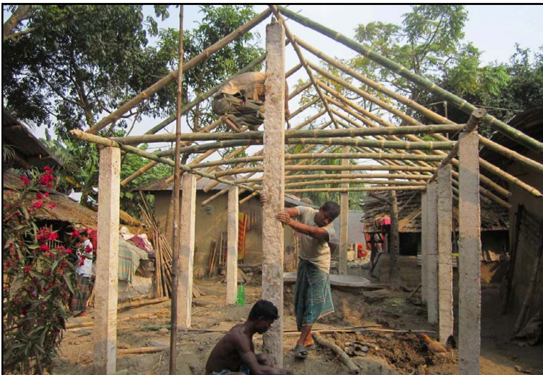
House Construction going on...
