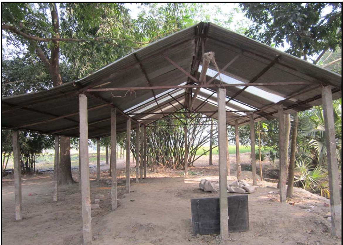
Jogahati Pr-school Construction Process in New Place...
