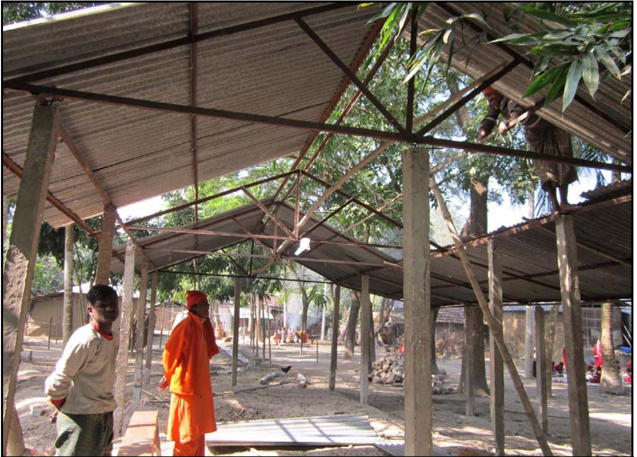
Jogahati Pr-school Construction Process in New Place...
