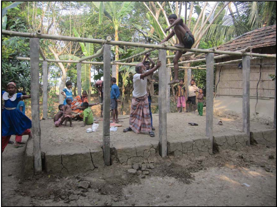
Construction of the Sorupdaho Study Centre...
