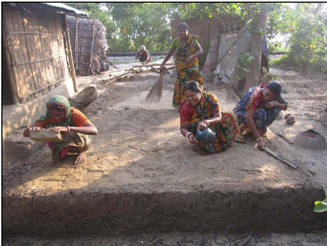
Moms Provides Physical Labour to Churamankati Tuition Study Centre Construction Process...
